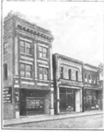
Home Office 525-7-9 N. 2nd St. Richmond, Va.
